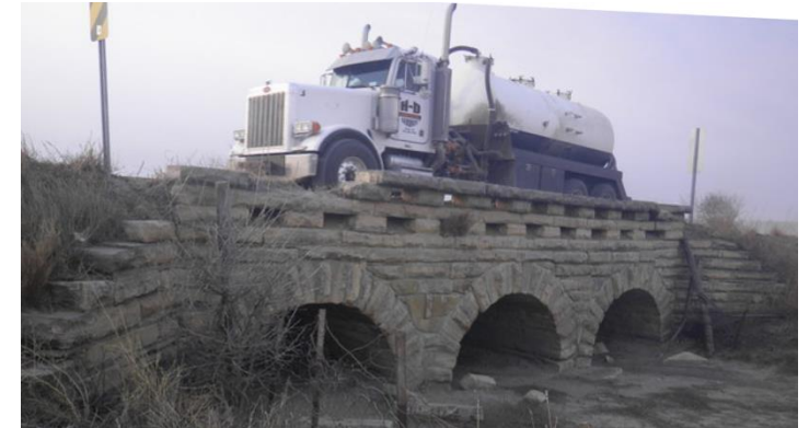
Ness County Stone Arch Bridge
